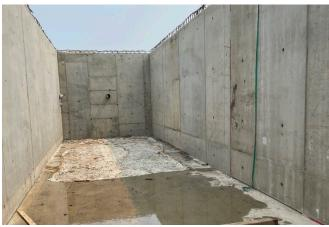
Admix C-500 was added to the concrete during batching for the foundations and apron. Xypex's crystalline technology ensures that microcracks up to 0.5 mm self-heal, significantly reducing maintenance costs and extending the structure's lifespan. Integrating Xypex Admix C-500 guarantees protection against water egress, even in extreme conditions, ensuring the reservoir's durability and operational efficiency for years to come.
